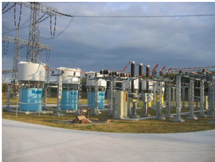
SEPS - Slovakia, Bratislava substation STUPAVA at 400/220 / 110kV shunt reactors and short circuit limiting reactors Phase I 90Mvar 10kV 5000A + 3 x + II stage 90Mvar
