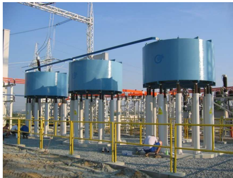
SEPS - Slovakia, Bratislava substation STUPAVA at 400/220 / 110kV shunt reactors and short circuit limiting reactors Phase I 90Mvar 10kV 5000A + 3 x + II stage 90Mvar
