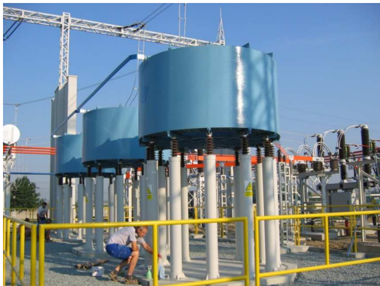
SEPS - Slovakia, Bratislava substation STUPAVA at 400/220 / 110kV shunt reactors and short circuit limiting reactors Phase I 90Mvar 10kV 5000A + 3 x + II stage 90Mvar
