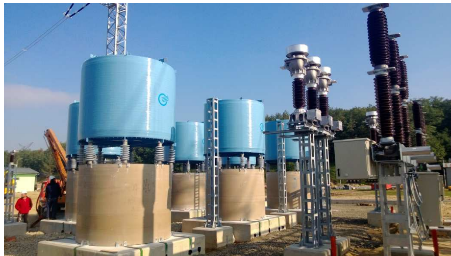
SEPS - Slovakia, Bratislava substation STUPAVA at 400/220 / 110kV shunt reactors and short circuit limiting reactors Phase I 90Mvar 10kV 5000A + 3 x + II stage 90Mvar
