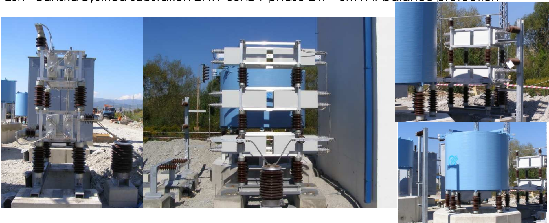
ZSR - Banska Bystrica substation 27kV 50Hz 1-phase 2 x + 6MVAR balance protection
