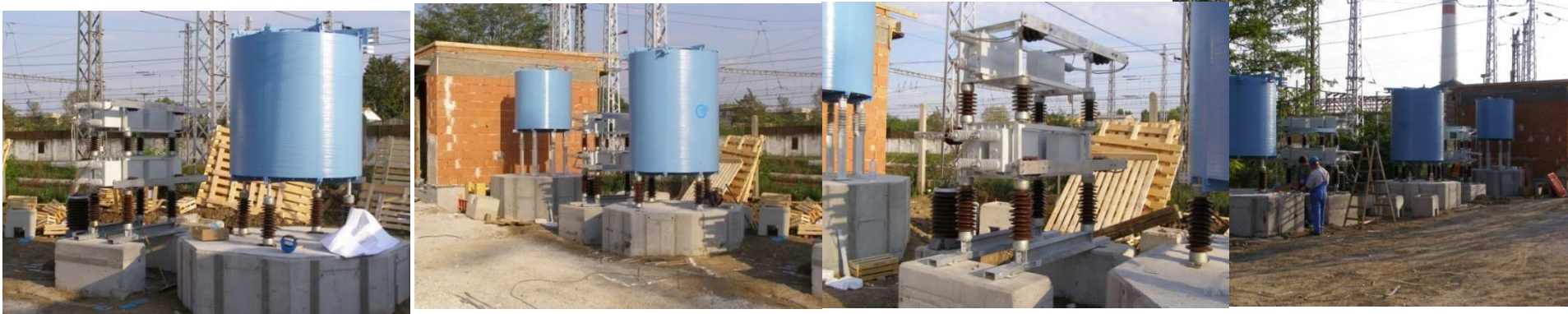
ZSR - Trnava substation 27kV 50Hz 1-phase 2 x + 6MVAR balance protection
